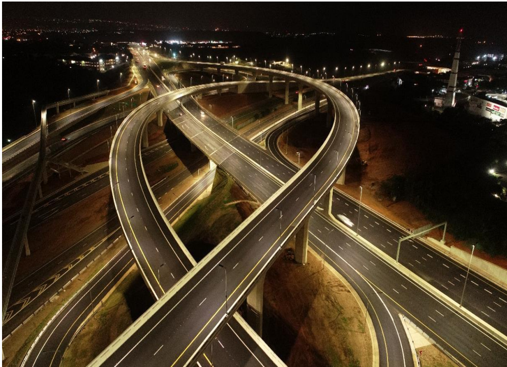
Mt Edgecombe Interchange (N2/M41), Kwa-Zulu Natal, South Africa 2018 – Prior to it being vandalised
